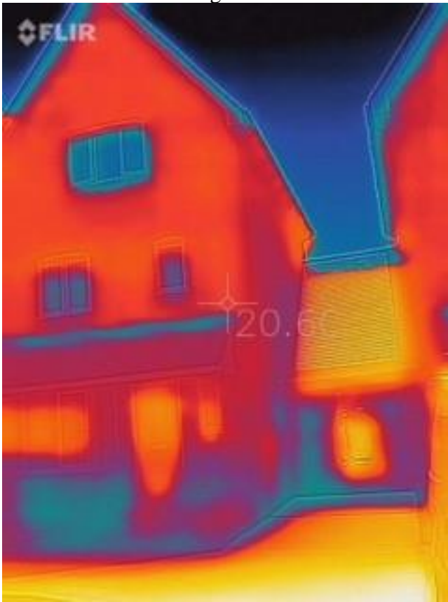
Front house-insulation good
